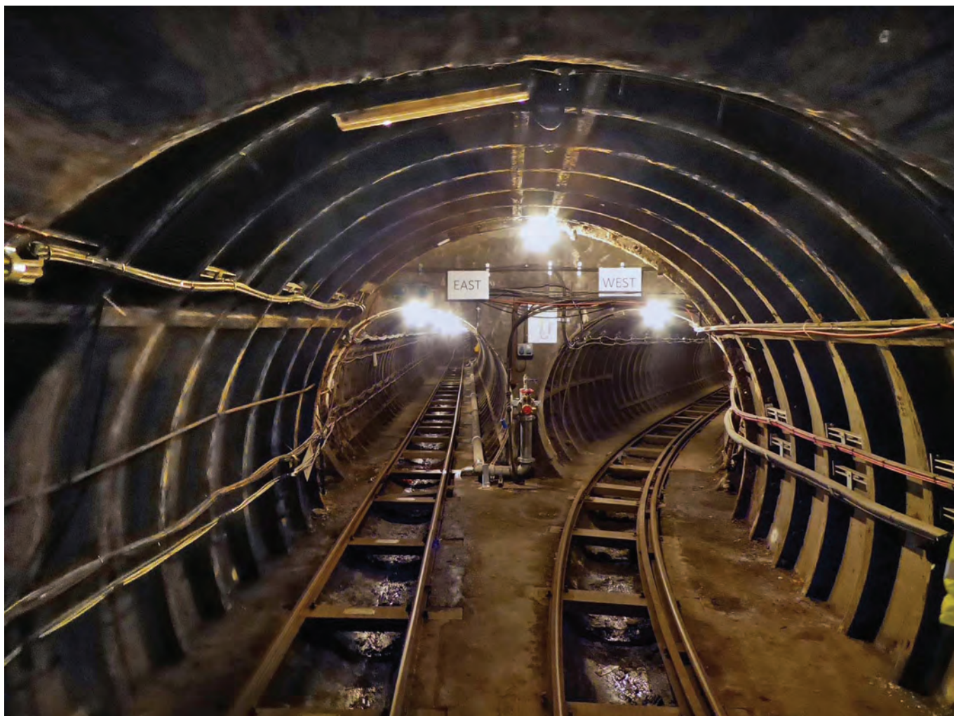
Junction at the bottom of the maintenance incline where the lines lead to the eastbound (left) and westbound platforms at Mount Pleasant
